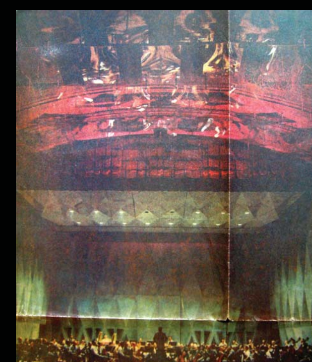
Figure 2: The world's first all-steel concert shell, complete with Plexiglas reflector panels over the proscenium, was installed in Northrop in 1961. The shell remained until 1969.
